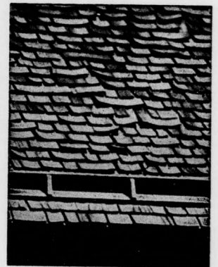
Wood Shingles After Five Years Wear
