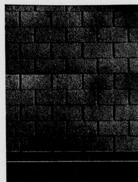
Reynolds Slate Shingles After Five Years Wear
