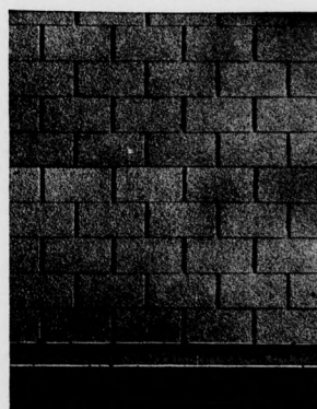
Reynolds Slate Shingles After Five Years Wear
