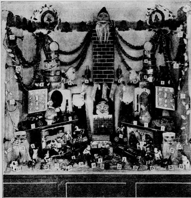
Photograph of Window Trim
