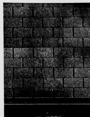
Reynolds Slate Shingles After Five Years Wear
