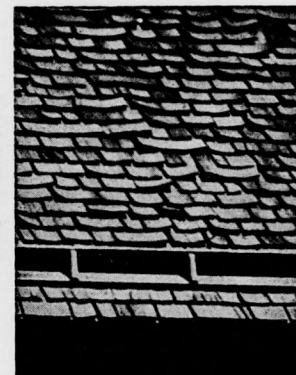
Wood Shingles After Five Years Wear
