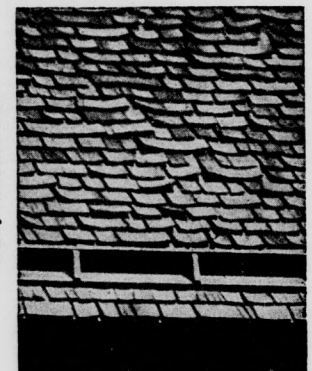
Wood Shingles After Five Years Wear
