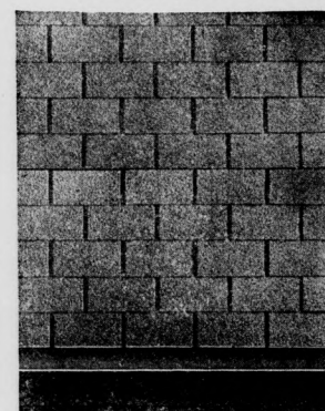
Reynolds Slate Shingles After Five Years Wear
