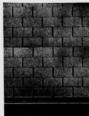
Reynolds Slate Shingles After Five Years Wear
