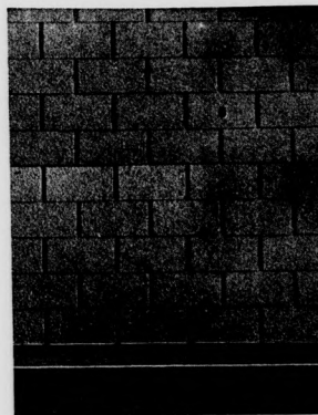
Reynolds Slate Shingles After Five Years Wear
