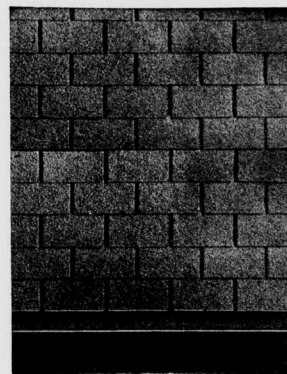
Reynolds Slate Shingles After Five Years Wear
