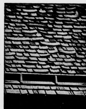
Wood Shingles After Five Years Wear
