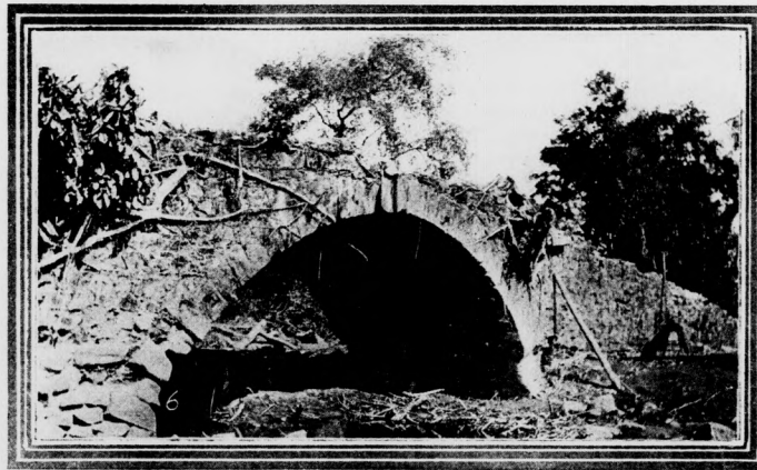
Bridge at Old Panama 400 Years Old.
