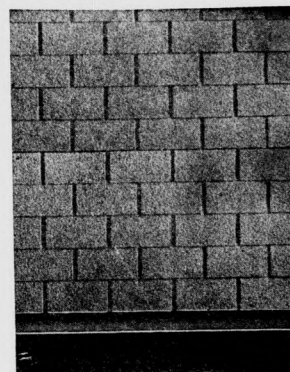
Reynolds Slate Shingles After Five Years Wear
