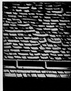
Wood Shingles After Five Years Wear
