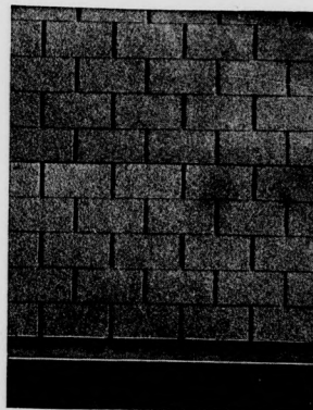
Reynolds Slate Shingles After Five Years Wear
