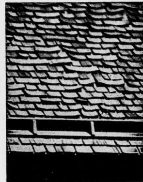
Wood Shingles After Five Years Wear
