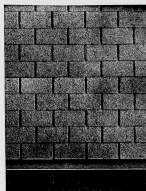
Reynolds Slate Shingles After Five Years Wear
