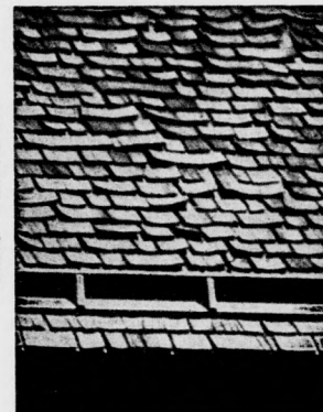
Wood Shingles After Five Years Wear
