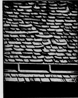
Wood Shingles After Five Years Wear
