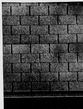
Reynolds Slate Shingles After Five Years' Wear
