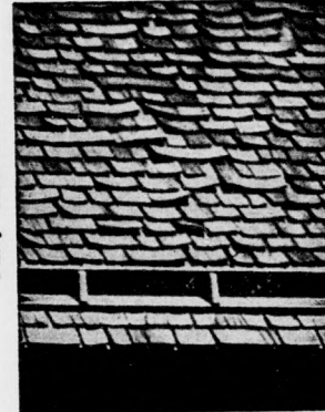
Wood Shingles After Five Years' Wear
