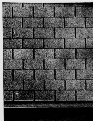
Reynolds Slate Shingles After Five Years Wear
