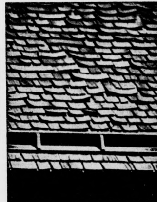
Wood Shingles After Five Years Wear
