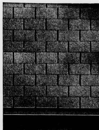
Reynolds Slate Shingles After Five Years Wear
