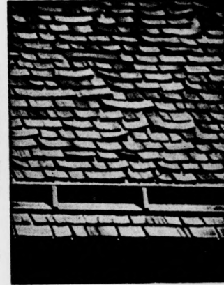
Wood Shingles After Five Years Wear
