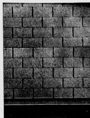
Reynolds Slate Shingles After Five Years Wear
