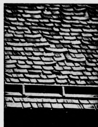
Wood Shingles After Five Years Wear
