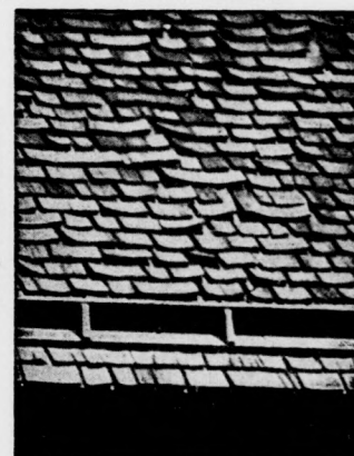
Wood Shingles After Five Years Wear
