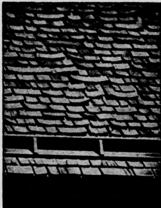
Wood Shingles After Five Years Wear
