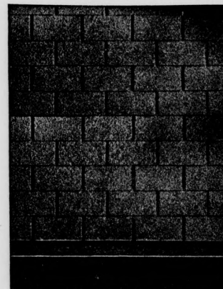
Reynolds Slate Shingles After Five Years Wear
