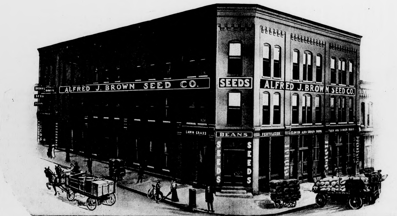
General Warehouse and Offices, Cor. Ottawa Ave. and Louis St.
