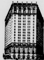
DETROIT 800 Rooms 800 Baths 200 room addition building
