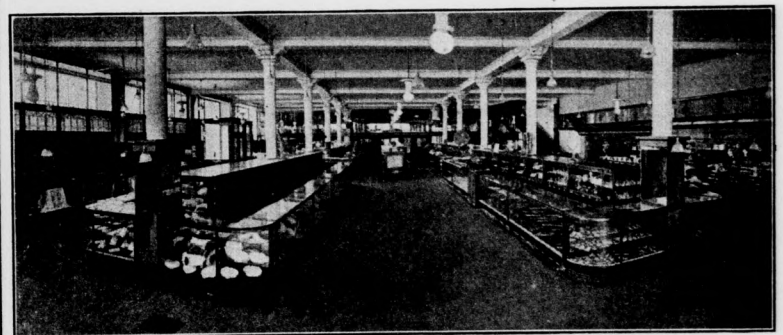
Wilmarth show cases and store fixtures in West Michigan's biggest store.
