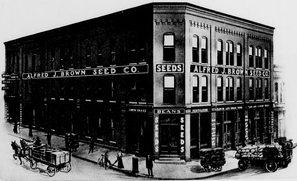
General Warehouse and Offices, Cor. Ottawa Ave. and Louis St.
