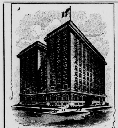
Five Stories Completed April, 1917
