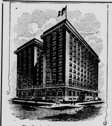
Five Stories Completed April, 1917
