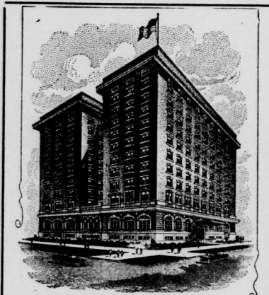
Five Stories Completed April, 1917
