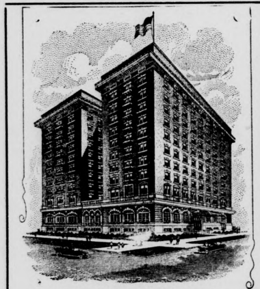
Five Stories Completed April, 1917
