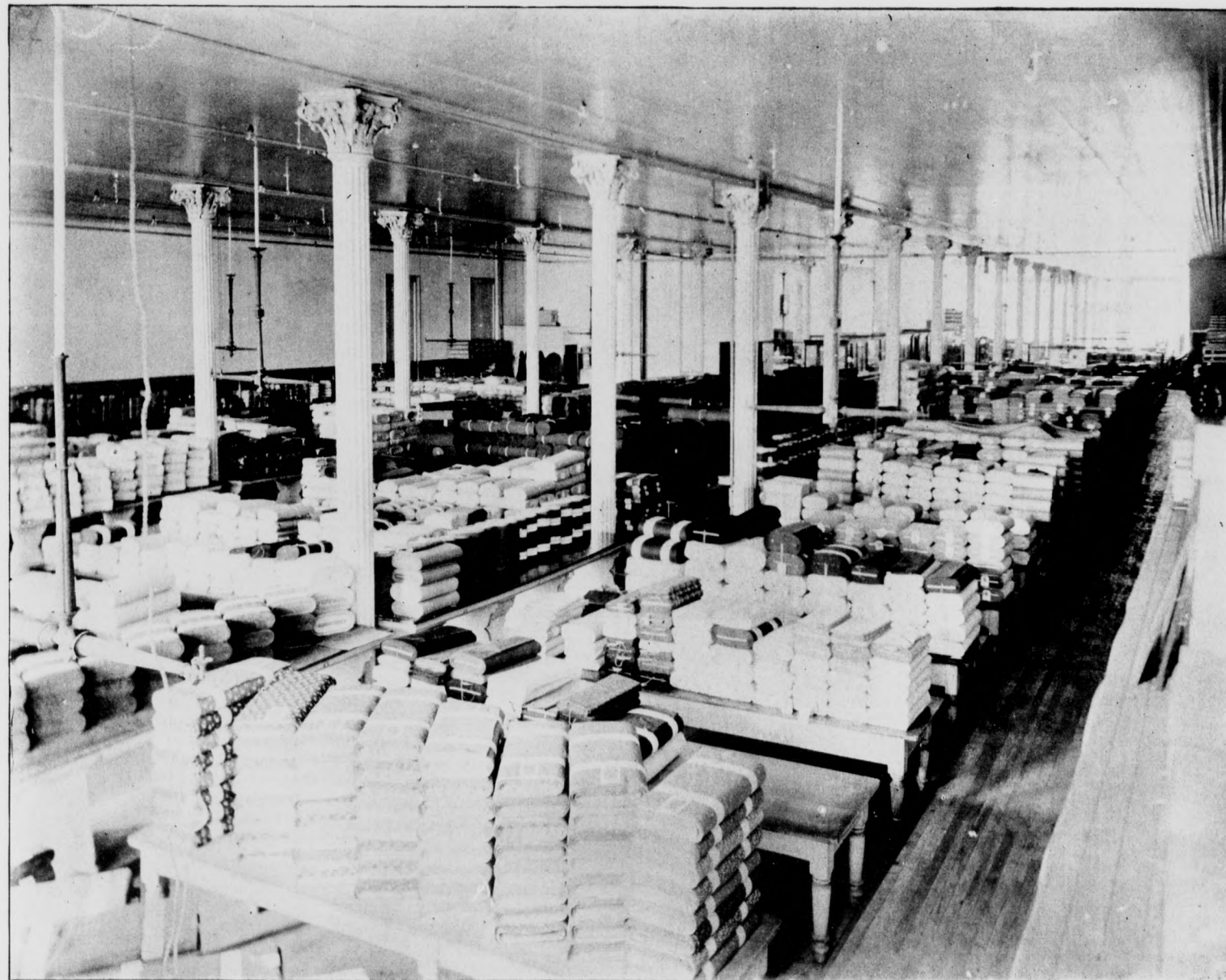
INTERIOR VIEW, FIRST FLOOR, 65 x 200 feet.
