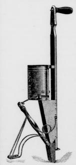
These Planters are fitted with Sheffield's famous patent adjustable seed disc, and spring brass cut-off. The disc revolves similar to the disc used in horse planters, and is the best finished and most accurate dropping disc ever used in corn planters of
