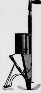
These Planters are fitted with Sheffield's famous patent adjustable seed disc, and spring brass cut-off. The disc revolves similar to the disc used in horse planters, and is the best finished and most accurate dropping disc ever used in corn planters of any description.
