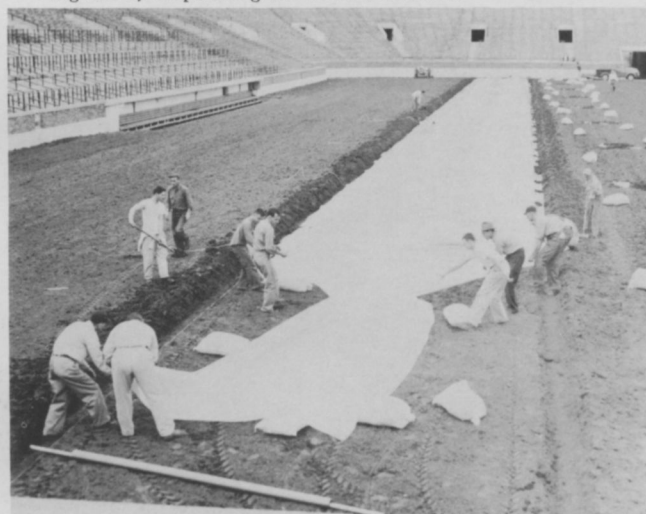
4 Placing plastic cover in position before covering edges with earth.
