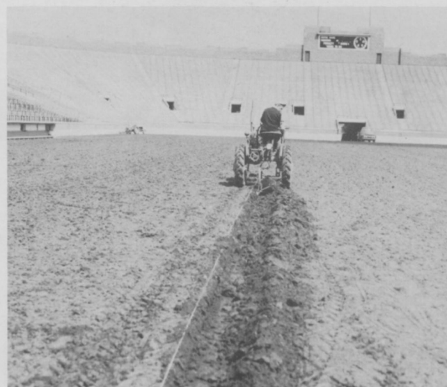
1 Tractor follows a guide line in digging trench which will hold and seal edges of tarpaulin.
