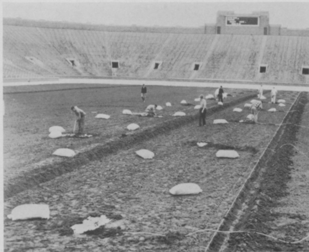
3 Straw pillows in place to hold up plastic tarpaulin. The cases on the pillows were of closely woven cotton to protect the plastic cover from being punctured by stiff straws.
