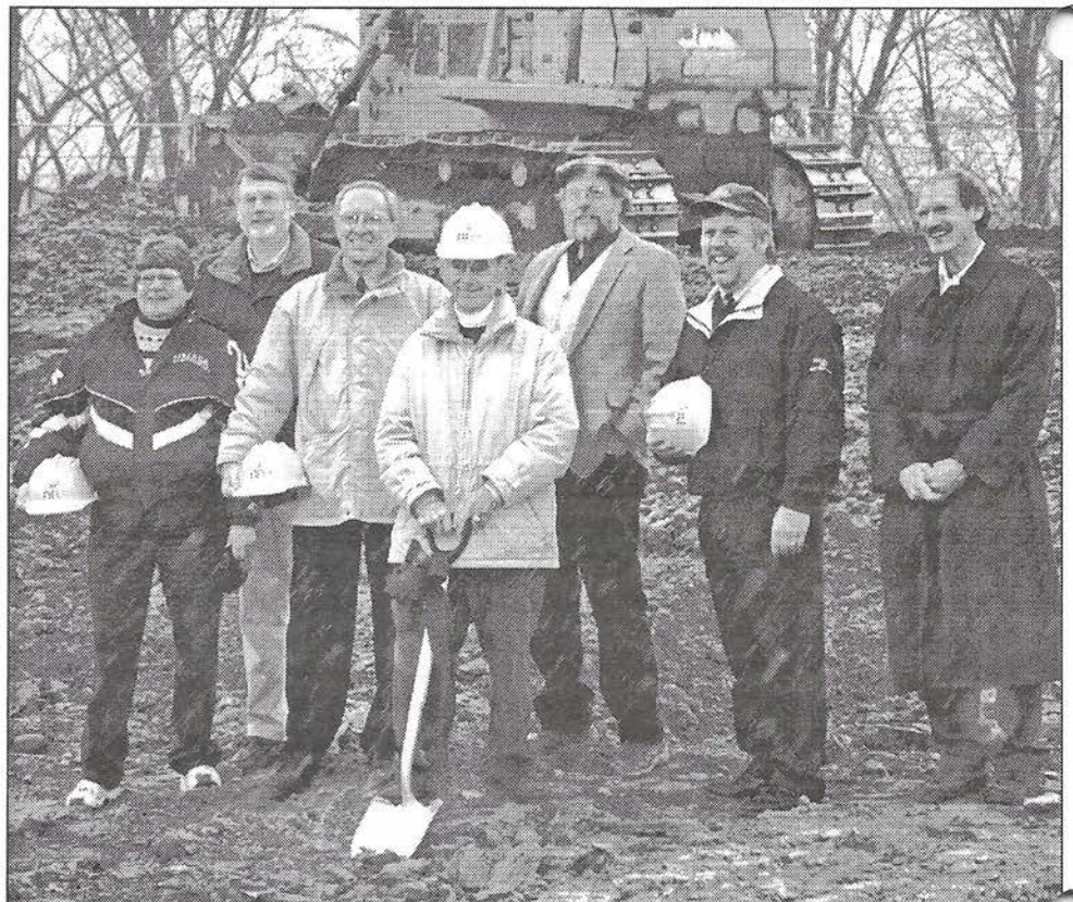
Pictured at the construction site on Jan. 6 are, l. to r.: Professor Pat Vittum; Peter Veneman, Plant, Soil, & Insect Sciences Department Head; Cleve Willis, Dean of the College of Natural Resources and the Environment at UMass-Amherst; Emeritus Professor Joseph Troll; Tom Griffin, Manager of the UMass-Amherst Turfgrass Facility; Gary Sykes, Executive Director of the New England Regional Turfgrass Foundation; and Professor Rob Wick. (Photo by Patricia Devine Cromack.)
