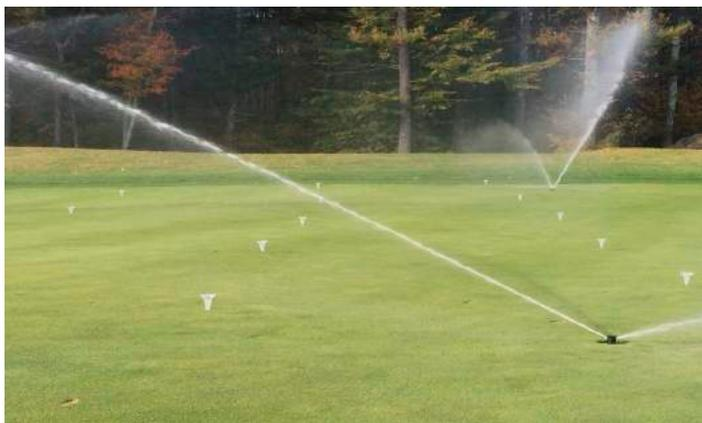
2. Whether you perform an audit or not, it's important to check the rotation of all rotors and ensure proper nozzle discharge. This is the year when any and all irrigation inefficiencies show up. A rotor not turning and clogged or incorrect nozzles will immediately show up as brown turf. Simply cleaning the pebbles from a clogged nozzle or inserting the proper nozzle to increase or decrease throw to the next rotor will significantly improve water coverage and distribution.
