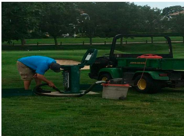
4. Clean all satellites and inspect all internal components for mice, ants, and spiders/cobwebs. Mice love to chew on wires and cables and ants find face plates to be very accommodating living quarters this time of year. Keeping your satellites free of these pests and their nests will increase the life span of your satellite components.
