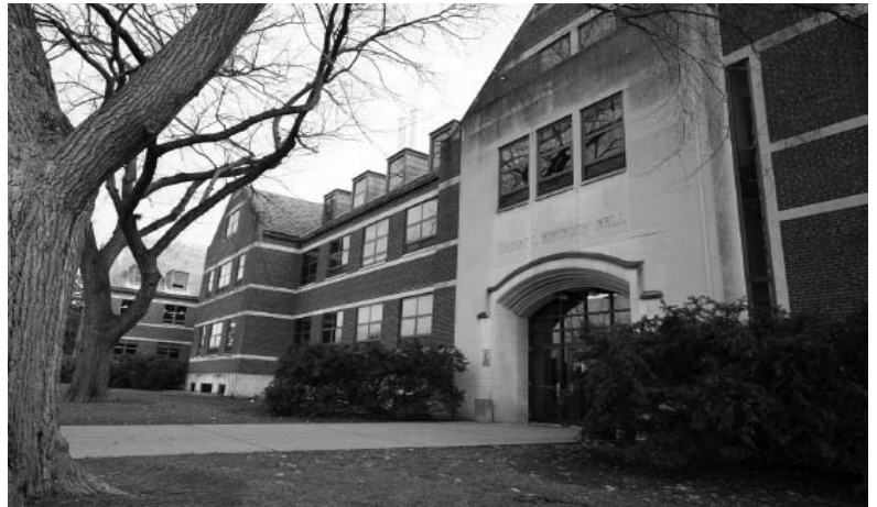
A photo of Anthony Hall, which was outfitted with Aircuity installations along with six other campus buildings.
