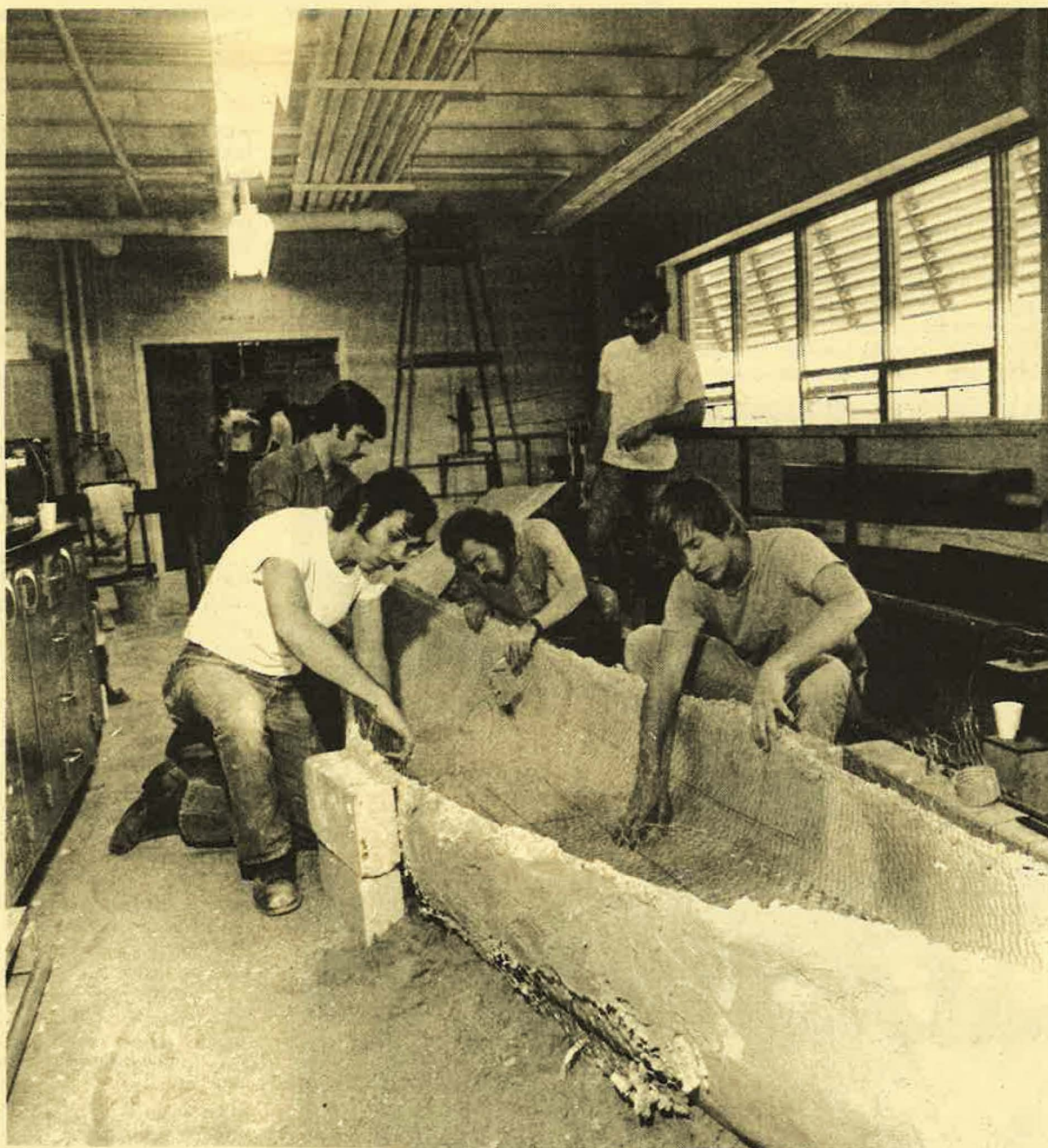
MSU juniors and seniors place chickenwire inside the plaster mold for the concrete canoe they plan to enter in the annual concrete canoe race to be staged Saturday (April 28) by Purdue University at Eagle Creek Park in Indianapolis. Working on the canoe, left to right, are Timothy Fox, junior from Detroit; Gary L. Boersen, junior from Jenison; Peter R. Wagoner, senior from Evart; and Robert W. Zuhl, junior from East Lansing. In the background is Michael B. LaFrance, junior from Lansing.
