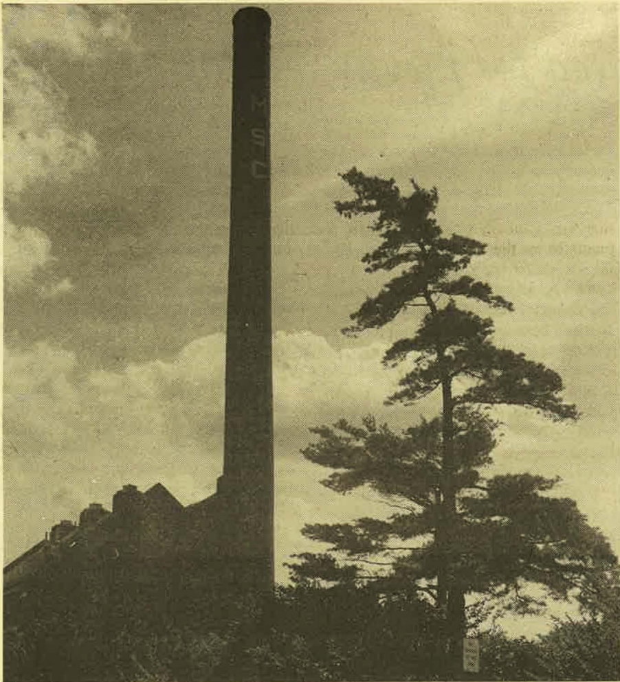
Shaw Lane power plant... photo by Dick Wesley
