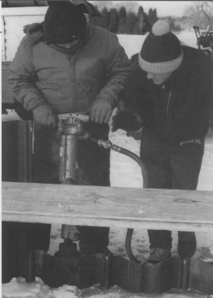
Steel seawall installed by Kurt Muendelein, Assistant Superintendent, and Dave Hinkle.
