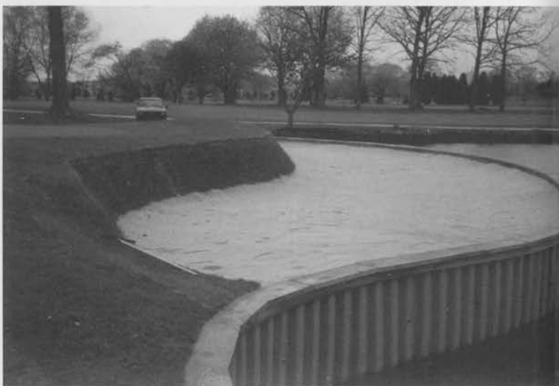
New PVC seawall installed behind #6 green.
