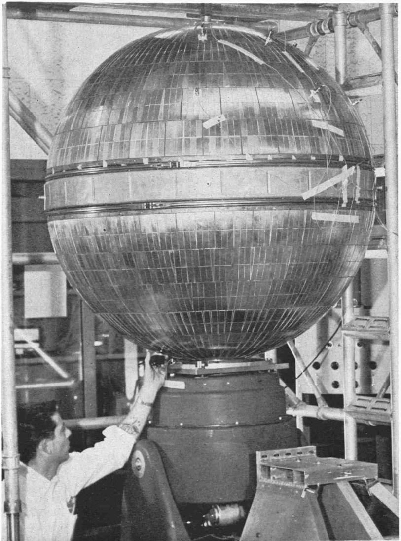
*The balanced and weighted model of the Courier is mounted on the vibration table to test its performance under the conditions which are encountered as the Thor-Able-Star accelerates the payload into orbit around the earth.*
