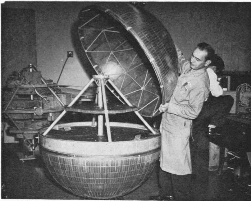
*Epoxy fiberglass shells are mounted on dummy structure to check fit of parts. Wooden mock ups are used to determine exact location of the 38 "black boxes" making up the Courier payload.*
