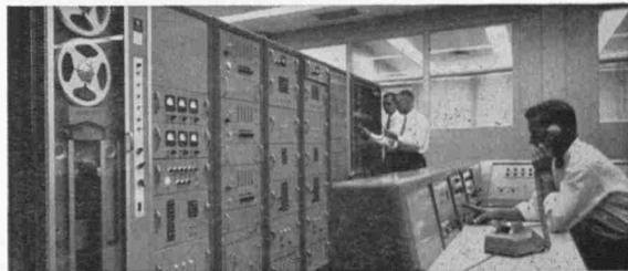
Representative of electronic aids functioning for P&WA engineers is this on-site data recording center which can provide automatically recorded and computed data simultaneously with the testing of an engine. This equipment is capable of recording 1,200 different values per second.
