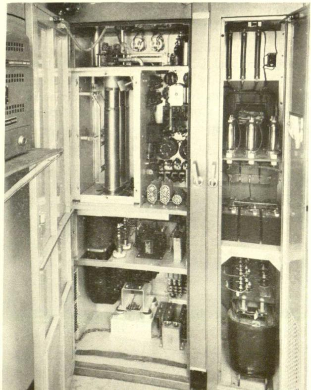
Rear view of the power amplifier and high voltage power supply. The final tank circuit with tubes in place can be seen in the enclosed box at the left. The unit on the left is the high voltage power supply.
