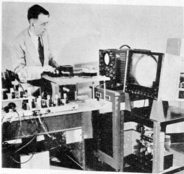
Principle elements of the sending terminal of the Ultrafax system.
