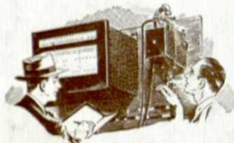
TYPICAL SOLUTION was development of first "turbidimeter," advancing work on water-purification equipment.
