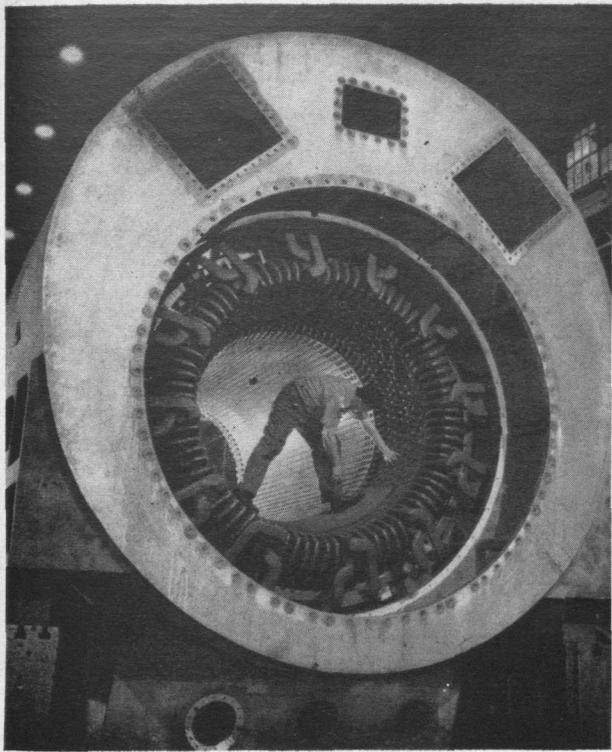
Inspecting one of the first turbine generators to be insulated with Thermalastic.
