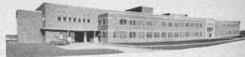
Pontiac's huge, new engineering building is one of the industry's most modern with every conceivable facility for designing better and better Pontiacs.
