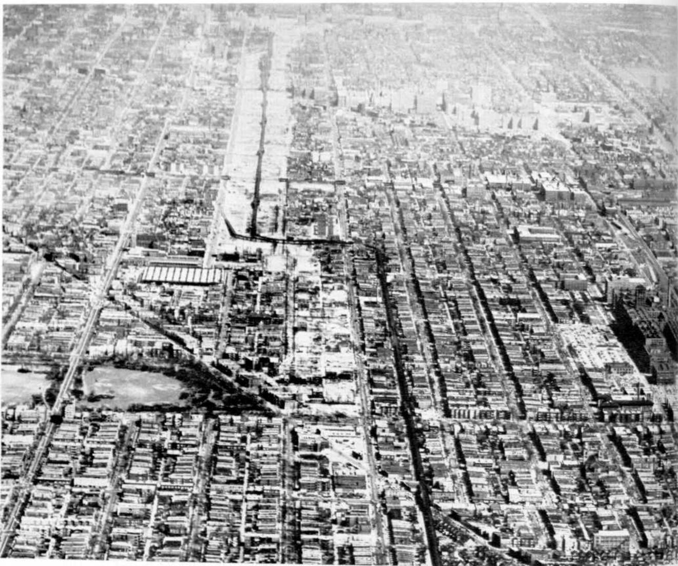
Photo taken during land clearance for Chicago's Congress Street Expressway shows some of the several hundred buildings that had to be removed for construction of this portion of the city's vital west side route.
