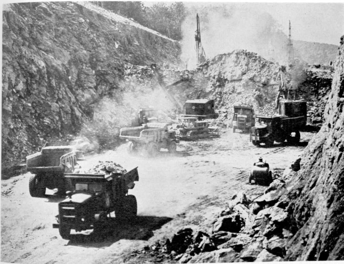
To reduce driving time and to produce the gentle curves and easy grades necessary for safe high-speed driving, today's roads are sometimes blasted right through hills rather than winding around them. Material removed from this hill of solid rock will be used to fill in nearby low areas.
